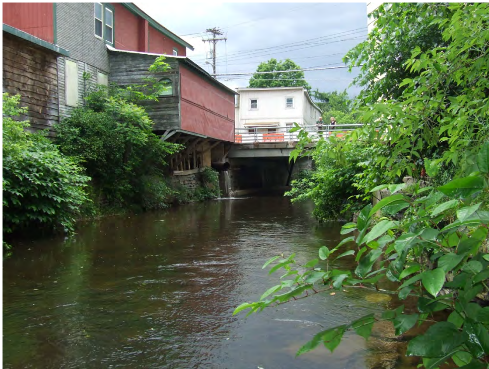
Figure 2.4: Looking downstream at the Main St. Bridge, an area normally impacted by flooding events.
