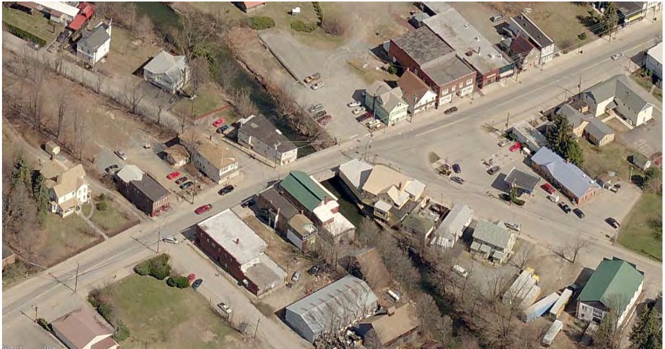
Figure 2.5: Aerial view of Main St. Bridge.
